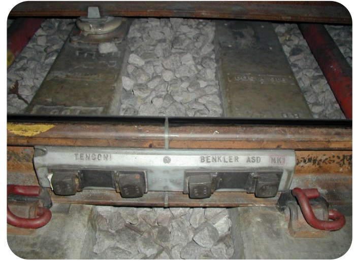
Insulated Rail Joints
